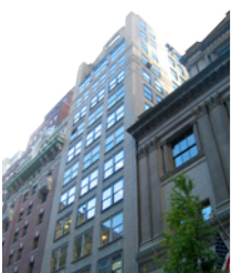
36 West 44th Street Between Fifth and Sixth Avenue
