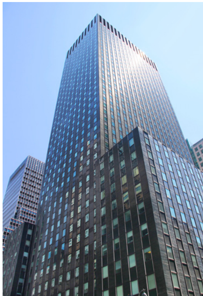
633 Third Avenue A premier one million square foot, class A office condominium building
